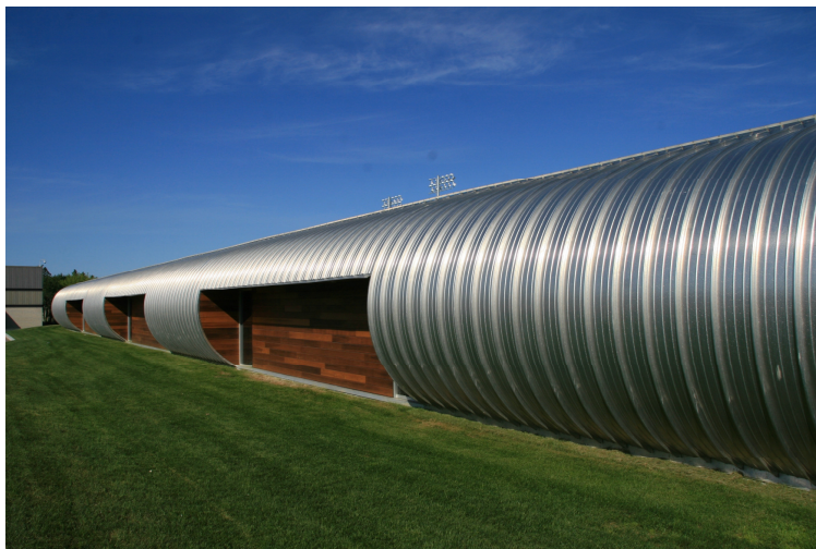
The University of Quebec's new arena features a distinctive, curved metal roof made with stucco embossed Kalzip 65/400 that extends down over one of the structure's walls.
